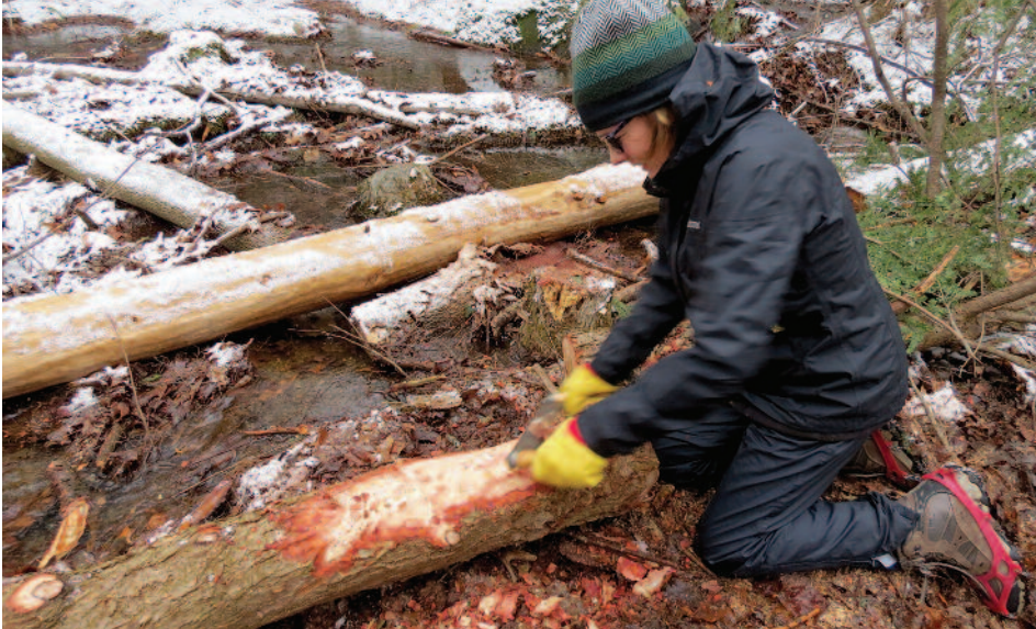
Volunteers help debark trees and build a footbridge at Basin Pond in Lee, and install bog bridging at Bob's Way in Monterey.
