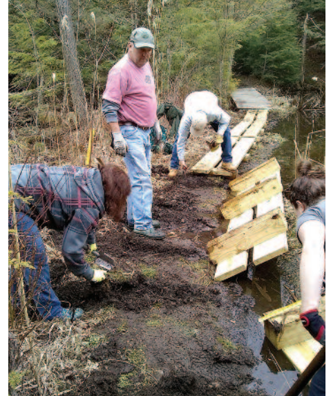
Volunteers help debark trees and build a footbridge at Basin Pond in Lee, and install bog bridging at Bob's Way in Monterey.
